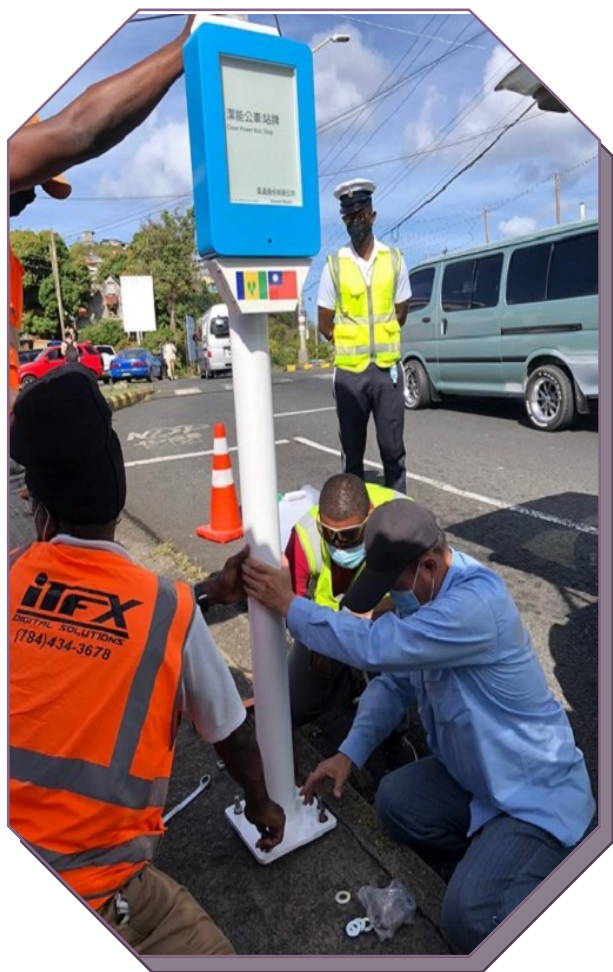
Installation of one of the bus management and monitoring systems being done by personnel from the ITSD, & ICDF and RSVGPF
