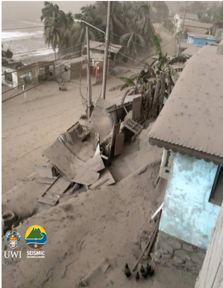
Photograph of collapsed structures due to the thick ash deposits from the explosions in early April 2021 at Soufrière St. Vincent.
